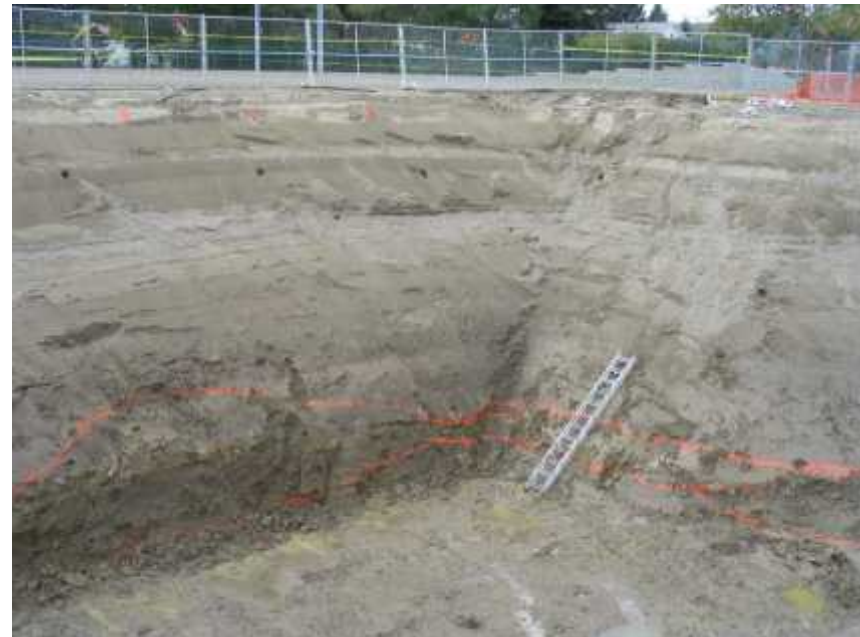
Secondary source removal to the east of Kal Tire
