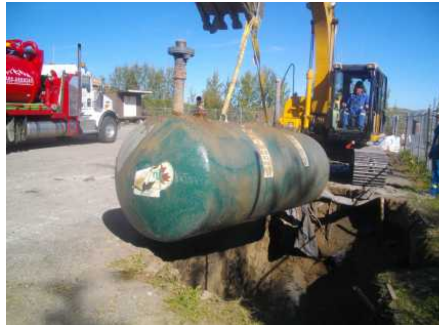
Example of an Underground Storage Tank Removal.
